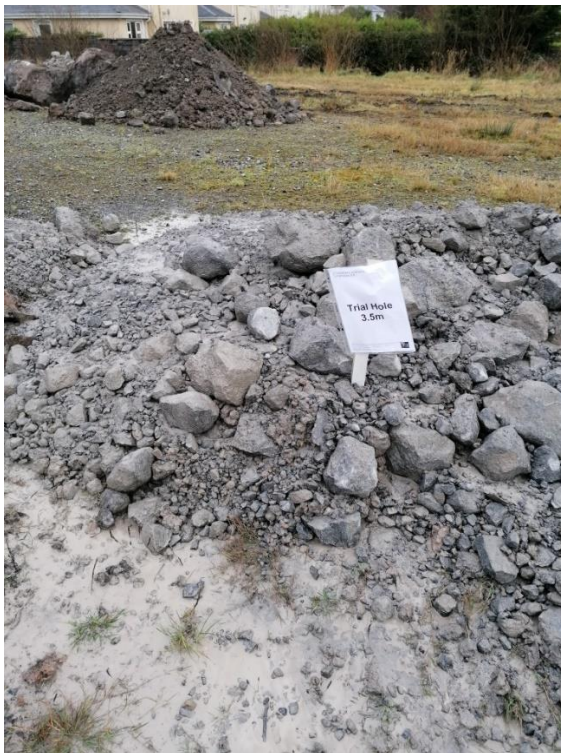
Figure 17: Trial Hole 3, 5m
